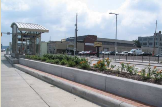
Euclid Corridor, Cleveland, OH 5,300 cubic meters of planting mix
